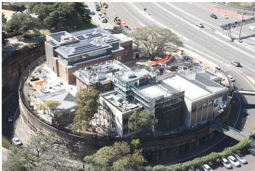
Fort Street Public School September 2023
